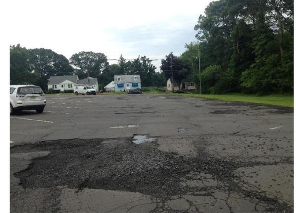
At the time of the assessment, the pavement throughout the school property was in deteriorating condition. Parking spaces can be replaced with pervious pavement to capture and infiltrate stormwater. The rear parking lot is receiving runoff from the roof in addition to the pavement. Installing pervious pavement can capture and infiltrate runoff. A preliminary soil assessment suggests that the soils have suitable drainage characteristics for green infrastructure.
