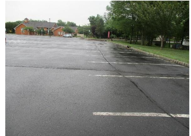
On the western end of the parcel, the site topography confirms runoff volume supply for two rain gardens that can capture, treat, and infiltrate runoff and one porous pavement section, which can manage additional stormwater. A preliminary soil assessment suggests that more soil testing would be required before determining the soil's suitability for green infrastructure.
