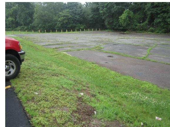
The turf grass area to the south of the parking garage appears feasible to construct a rain garden to receive runoff from a portion of the western parking lot. This green infrastructure practice will capture, treat, and infiltrate stormwater. A preliminary soil assessment suggests that the soils have suitable drainage characteristics for green infrastructure.
