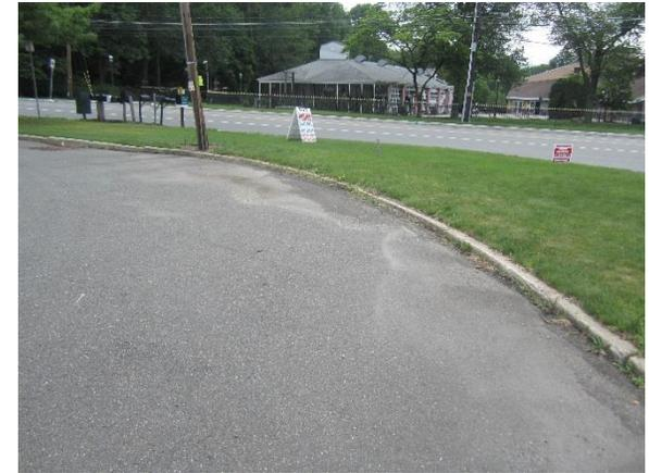
Two grassed islands at the parking lot entrance can be converted into rain gardens to help manage stormwater. These rain gardens will be aesthetically pleasing while capturing, treating, and infiltrating runoff. Parking spaces can be replaced with pervious pavement to capture and infiltrate stormwater. A preliminary soil assessment suggests that the soils have suitable drainage characteristics for green infrastructure.
