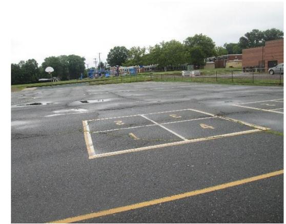
Parking spaces can be replaced with pervious pavement to capture and infiltrate stormwater. The paved play area to the west of the school can also be converted to pervious pavement to provide additional runoff an opportunity to infiltrate. Two bioretention systems can be installed to capture, treat, and infiltrate rooftop runoff. A preliminary soil assessment suggests that the soils have suitable drainage characteristics for green infrastructure.
