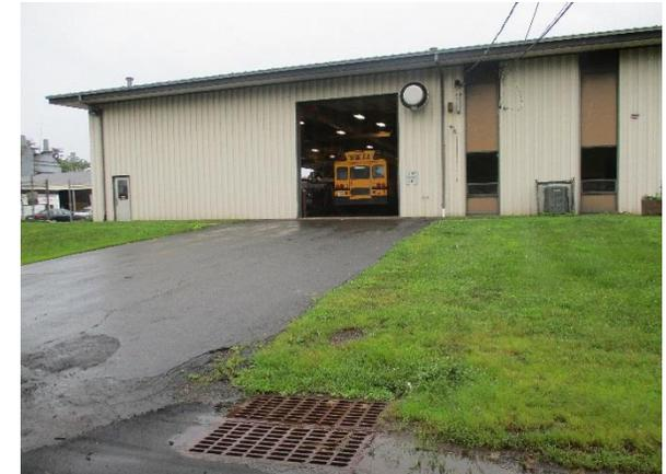
Parking spaces can be replaced with pervious pavement to capture and infiltrate stormwater. A bioretention system can be installed to capture, treat, and infiltrate rooftop runoff. A preliminary soil assessment suggests that the soils have suitable drainage characteristics for green infrastructure.
